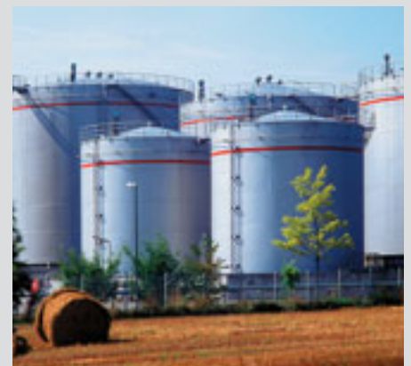
Industrial steel constructions
