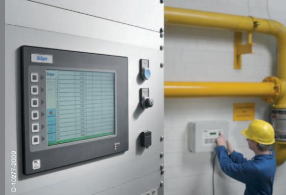
The Dräger REGARD 3900 Modbus Gateway is required to enable communication between the Dräger REGARD 3900/3910 and Dräger RVP 3900 visualisation panel. The data which is made available by the gateway contains all of the real time gas levels and alarm status of each of the connected control systems. For
