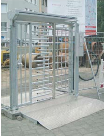
Turnstile on mobile stand with integrated door for temporary protection of a construction site
