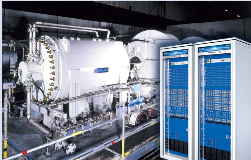
Turbomachinery test facility at Siemens, Duisburg/Germany
